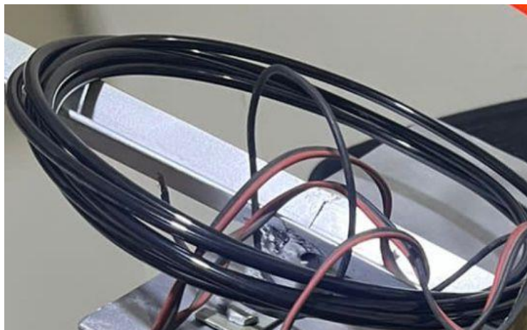
Figure 17: Hoses Source: self made
